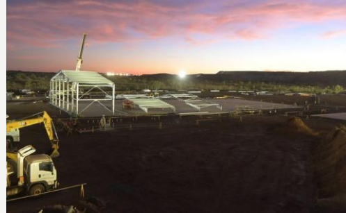
Industrial Warehouse Pilgangoora, Pilbara Large-span warehouse supporting a major resources operation.
