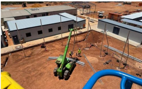
Remote Housing Packages Leonora & Lamington Remote and regional housing delivery with TR Homes / MRN.
