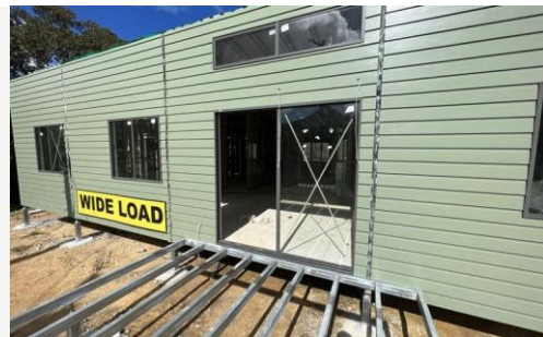
Modular Housing Program Regional NSW ~10 modular homes delivered fast-tracked for bushfire relief.
