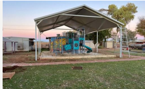
Remote Community Schools Central Desert WA School builds and upgrades across remote communities.
