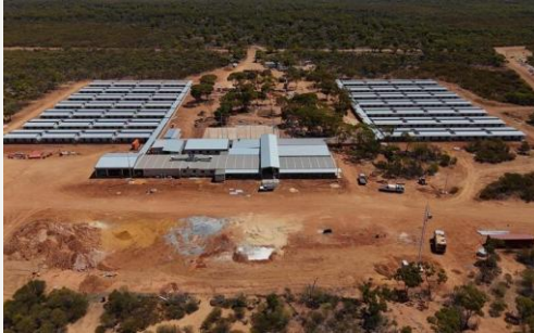
Remote Workers' Camp Mid West WA Accommodation camp build and fit-out in a remote, logistics-heavy location.
