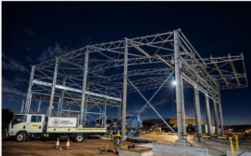
Workshop Build Aurenne, Regional WA Purpose-built workshop — structure and coordinated services.
